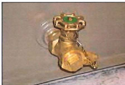
Figure 3. Drain valve with sampler.
