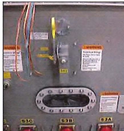
Figure 8. VFI transformer with visible break.
