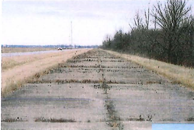
Existing Unused Route 66 Slab Segment (Representative Condition)
