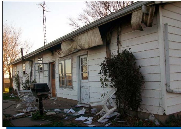
On November 17, 2013 a thunderstorm with damaging winds near Nokomis knocked down a power pole causing a line connected to a house to spark in the attic causing a house fire.
