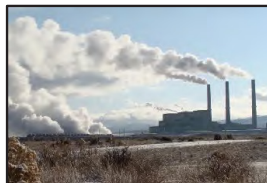
Coal Burning Power Plant
