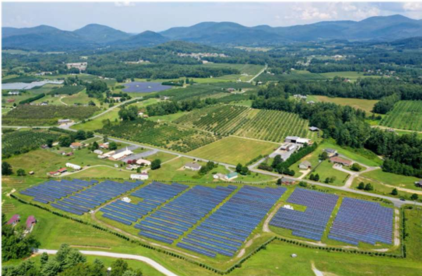
IS16 is a 3MW solar facility in Henderson County, NC. In 2021, this solar facility produced enough energy to offset the carbon dioxide emissions of almost 600 cars on the road
