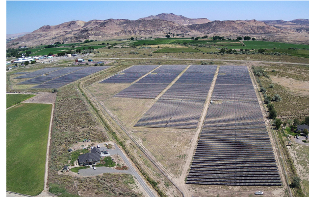
▲ Vale Air, Oregon, 13MW
