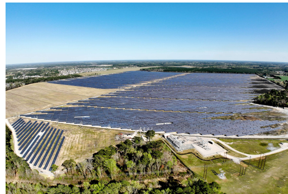
▲ Innovative Solar 46, North Carolina, 100MW
