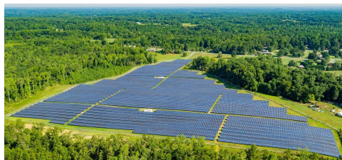
Charlie 6MW in Guilford County, NC
